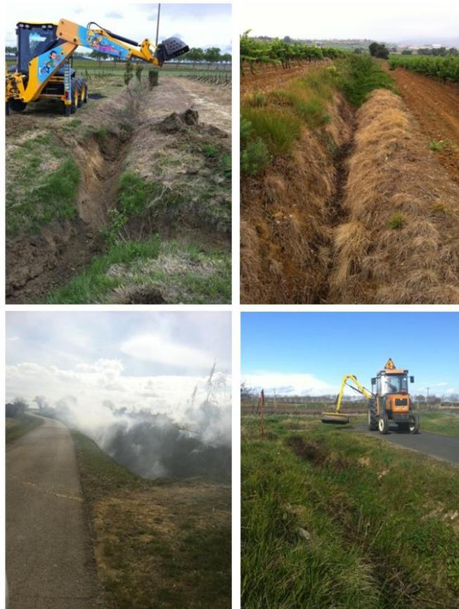
**Figure 1.1: Ditch maintenance.** Ditch maintenance is a combination and a succession in time of four basic operations namely dredging, mowing, chemical weeding and burning. On top: dredging on the left and chemical weeding on the right. On the bottom: burning on the left and mowing on the right.
